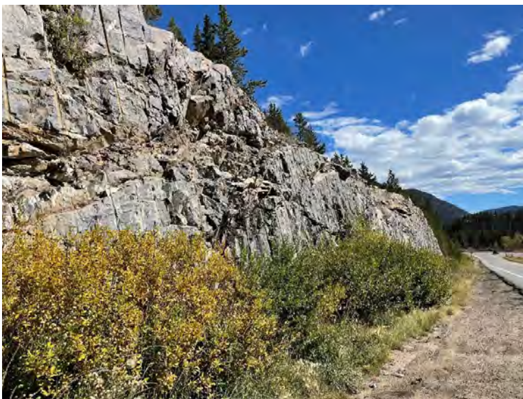
Figure 71. Bakerville exit presplit rockcut
