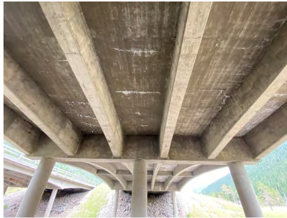
Figure 31. General view of the underside of the deck in Span 1
