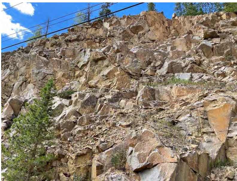
Figure 72. US 6 cushion blast type rockcut
