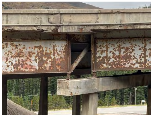
Figure 15. Typical condition of movable bearings, Pier 2 Girder A
