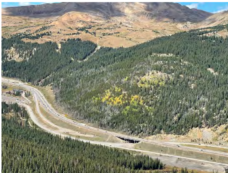
Figure 70. Aerial view from US 6 interchange of landslide area above I-70 (MP 215.5 to 216.4)
