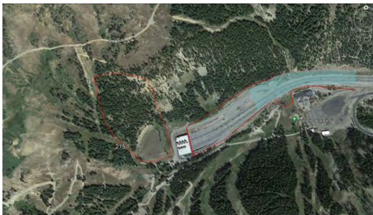
Figure 68. Historic EJMT landslide area and buttress located at MP 215
