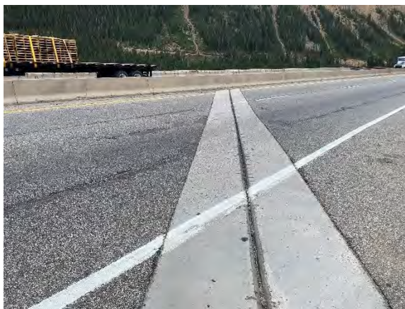
Figure 9. Expansion joint at Pier 2
