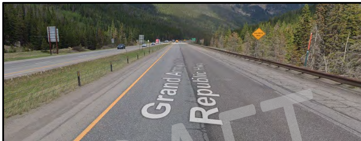
Figure 1: Typical View Eastbound, I-70 MP 215.30-221.50
