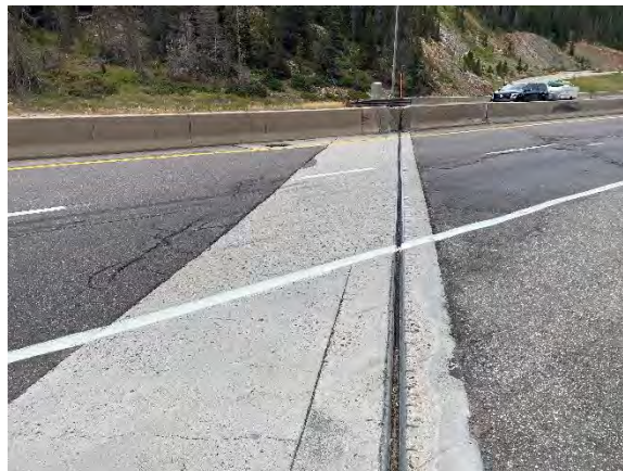
Figure 21. Expansion joint at Abutment 1
