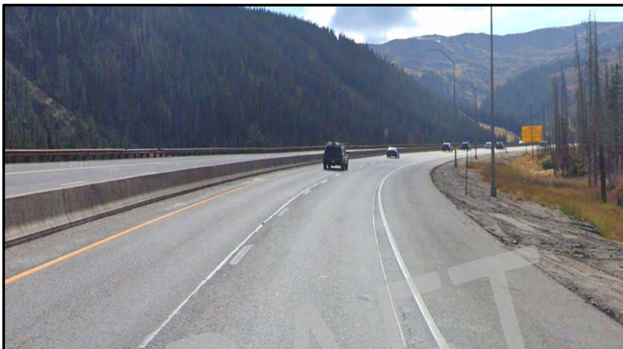
Figure 38: View approaching tunnel near MP 216 Westbound I-70 Segment 2
